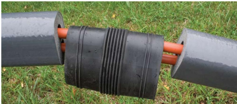
With one person holding the pex pipes, the second person can slide the third 8 foot piece of MAXX-R insulation all the way to the other end butting against the boot and first 2 sections of MAXX-R insulation. This will help straighten the pipes and make your installation easier.
