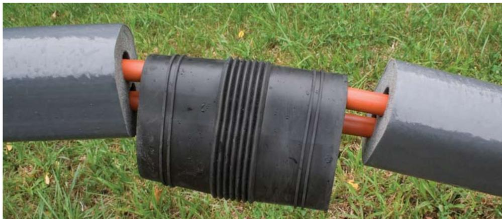
With one person holding the pex pipes, the second person can slide the third 8 foot piece of MAXX-R insulation all the way to the other end butting against the boot and first 2 sections of MAXX-R insulation. This will help straighten the pipes and make your installation easier.
